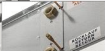
Anti-twist device
